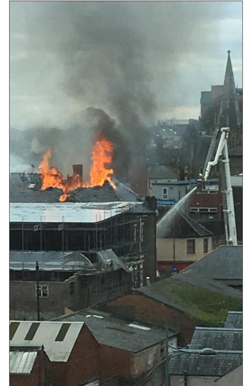
FLAMES: The March 2018 Drill Hall fire. Picture: Jonathan Jones
