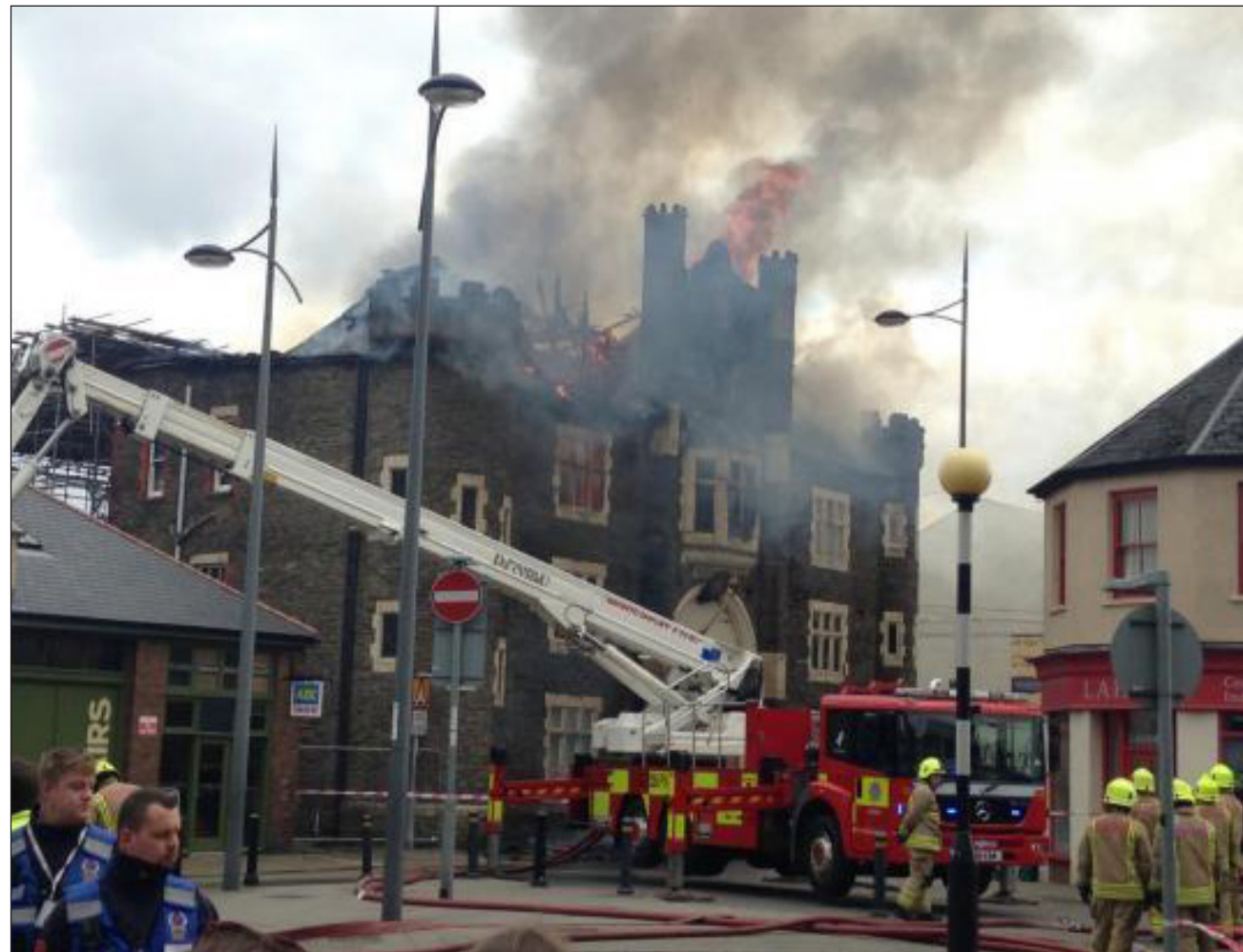
BLAZE: Flames leap from the well-aight Abundant Life Centre building in Lower Dock Street, Newport.
